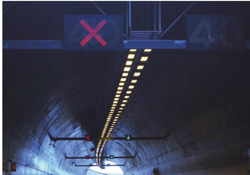
**SCANLIGHT** is a Dimmable Addressable lighting control system developed specifically for Road Tunnel Applications to economically deliver optimum lighting conditions best matching the Luminance Reduction Curve, with performance far exceeding conventional or switched stage systems, and capital and running costs substantially lower than conventional switched systems. **SCANLIGHT** offers the following benefits:
